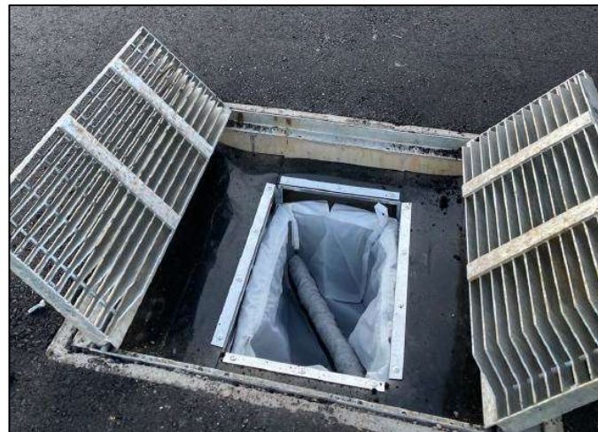
Figure 6.3: Installed Oil Sock
